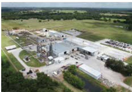
Callidus 82,000 sq. ft. manufacturing and fabrication facility in USA
